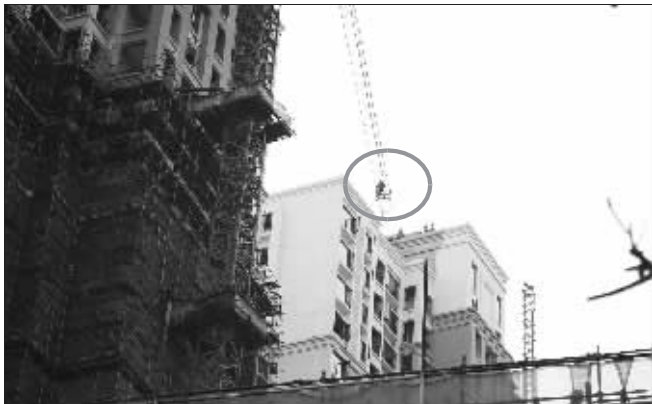
讨薪民工站在塔吊吊臂顶端
